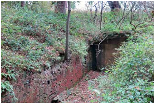
Welbeck Abbey: the eastern portal of the tunnel shown on the OS map, where it opens into a cutting on the west side of the Burial Ground Plantation. Photo Clive Penfold
